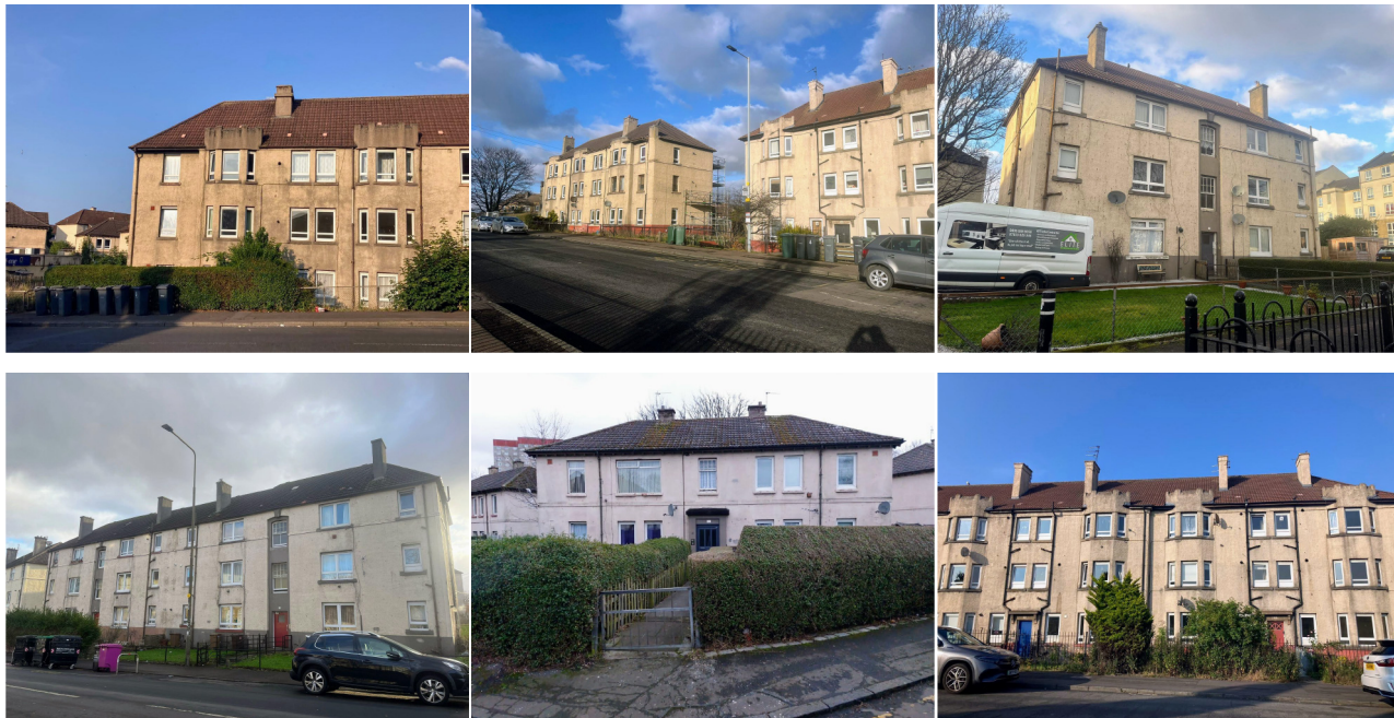
Examples of Lochend housing blocks due for work under the MTIS programme.
